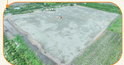
Wastewater Treatment Plant Sand filling (completed) Pile pressing (in progress)
