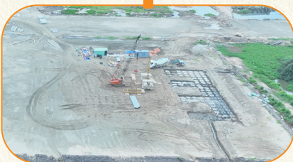
Water Supply Plant Sand filling (completed) Pile pressing (in progress)
