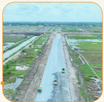
DD3 Road Roadbed compaction (in progress)
